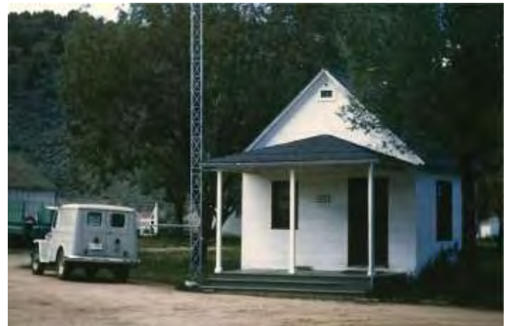
Bridgeport Ranger Station office building, Toiyabe National Forest, four miles northwest of Bridgeport, California, on U.S. Highway 395, 1933-1962.
