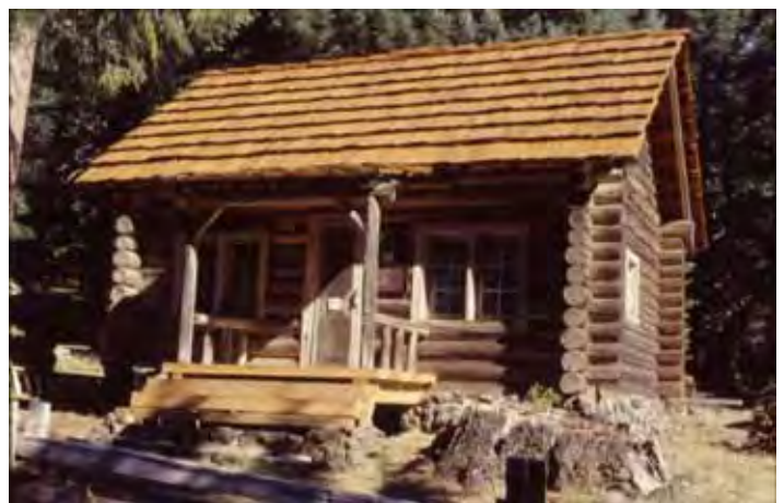
Fish Lake Ranger Station dispatcher's office cabin in 1926 (top) and after recent renovation of roof and porch (bottom).
