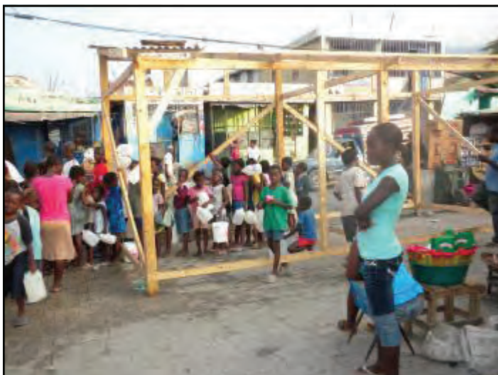
A prototype of a wood-frame temporary shelter is inspected on a street by young Haitians who will benefit from the project.
