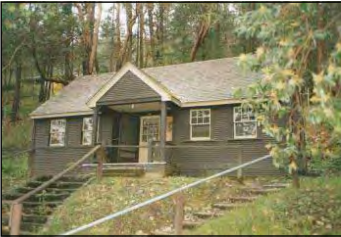
The old Star Ranger Station office across Upper Applegate Road from the current office and old 1911-1914 historic office.
