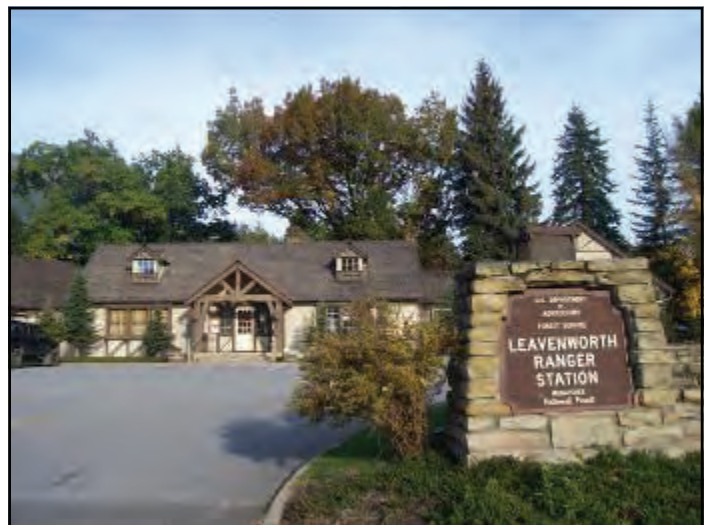
The historic Leavenworth Ranger Station office today.
